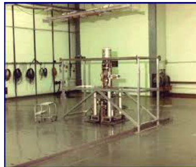
Figure 2. The Fast Burst Reactor Facility
